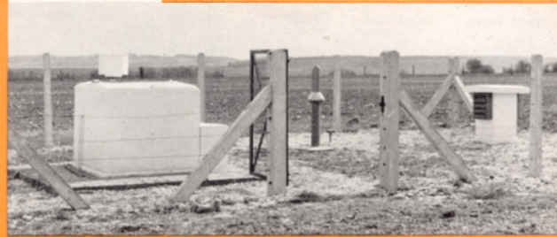
Observer Post No. 4 showing (left to right) entrance turret with GZI, Survey Meter Probe, BPI Baffle and ventilation turret
