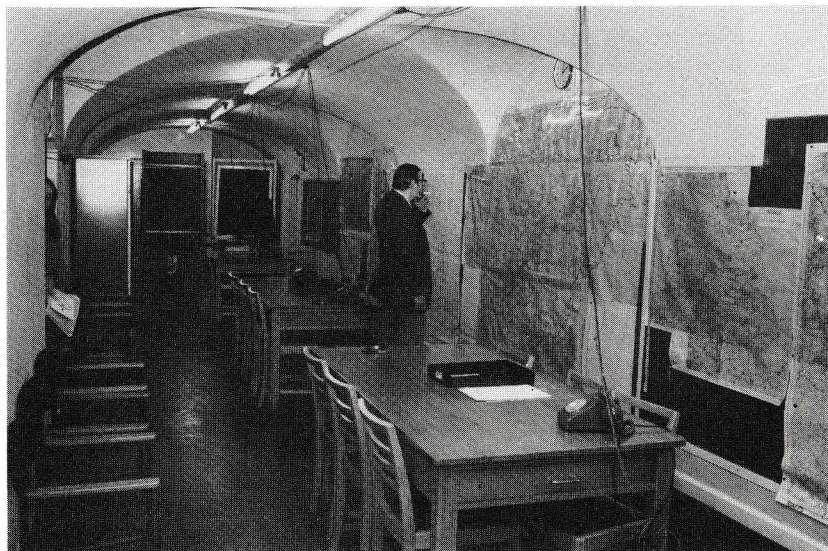
Members of the public visiting the bunker underneath Cusworth Hall, near Doncaster. This is one of two County Emergency HQs – the other is under County Hall in Barnsley. Martin Jenkinson
